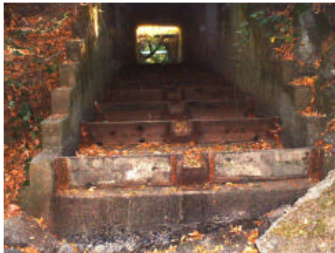
These wooden baffles leak and trap hundreds of juvenile salmonids each spring.
